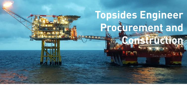
ODE acted as Design subcontractor under BiFab, who acted as Topsides EPC contractor, for this West of Shetland facility. The field design consisted of four subsea wells (two producers and two injectors) tied-back to a topsides processing facility on a single slim jacket installation, with produced oil stored in a subsea storage tank for shuttle tanker offloading via a single anchor loading (SAL) System.
