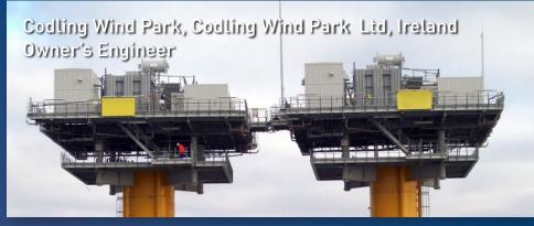
Concept and feasibility development of the WTG foundations, onshore and offshore substation, and array cables. Also providing wider technical expertise as necessary to project.
