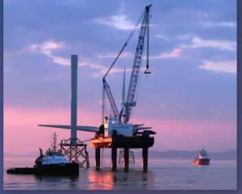
First full-field offshore wind farm development deploying jacket WTG foundations and large 5MW turbine. Project management contractor overseeing conceptual studies, FEED, detailed design etc.
